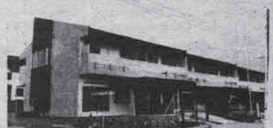
"SEA-HILL" 2-Storey Split-level Terrace House. Ground floor: Lounge, dining room, kitchen, servant's quarters, bathroom, car porch, spacious front and rear gardens. First floor: 3 bedrooms, 2 bathrooms, family hall, front and rear balconies.
